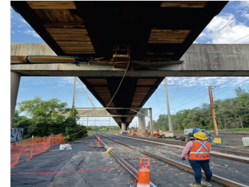
Track and Structures Rehabilitation
