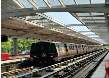
Railcars & Railcar Facilities
