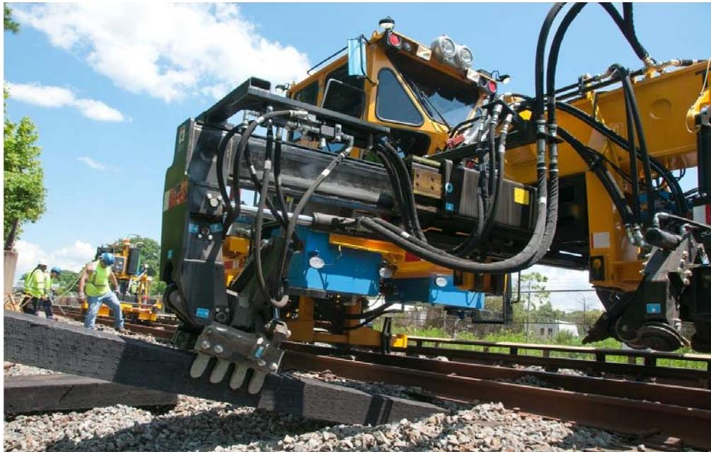
Photo of Track maintenance crew replacing ties on track number 1 between Rockville and Shady Grove using the recently delivered Tie Inserter
